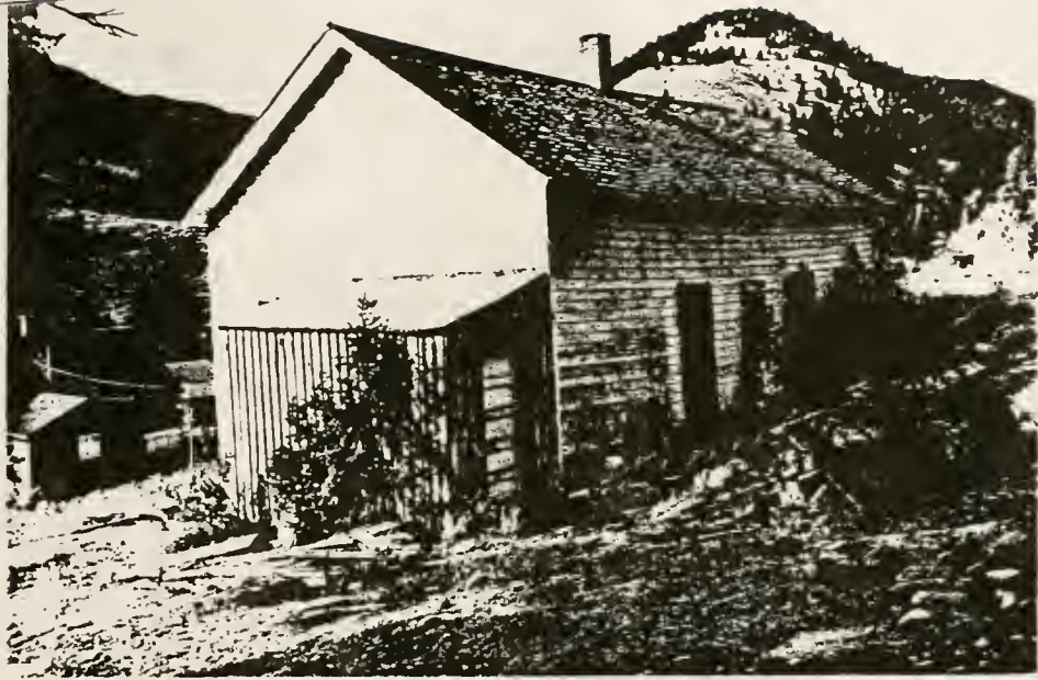
Figure 202. Jardine school house (Structure #79), north view.
